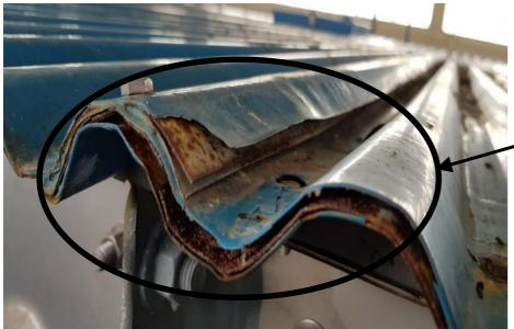
Corroded corrugated epoxybonded galvanised roof cover with gaps of stainless steel water tank body.
