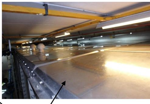
Full stainless steel water tank (i.e. tank body, drainage panel, bottom panel and tank roof cover shall be of grade 316 or better).
